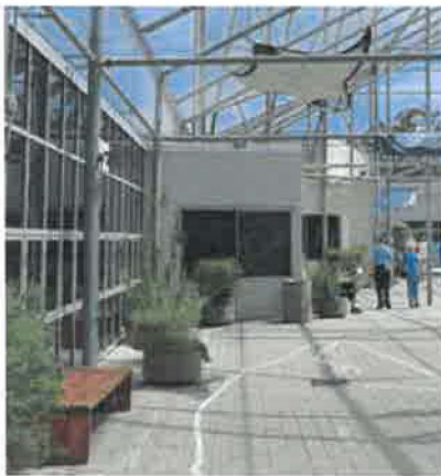
Windows into the sales area (currently offices) will attract visitors who are resting in the courtyard.
