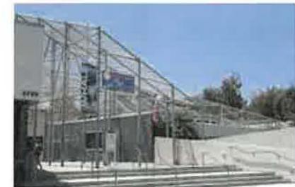
Chain link fencing and corrugated metal siding are important architectural features of the Gehry design.
